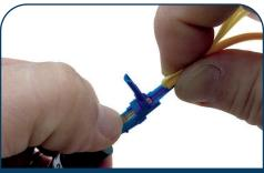
7. Slide activator tab towards connector tip. Remove from VFL. Ensure fiber is straight, hold Kevlar to one side (2.0mm seat tube at rear of connector). Close hinge.
