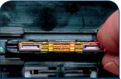
12. Insert the right fiber forward into splice, watching for movement of the left fiber as it is pushed from within the splice and/or loss of light if using a VFL.
