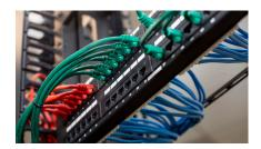
Patch cables that feature snagless boots to prevent tangles when pulling through openings, RJ45 clip locks to prevent accidental disconnects, and bandwidth up to 10Gbps.
