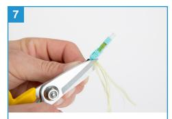
Thread the connector boot on enough to catch the Kevlar strands, then trim the strands and thread the boot on the rest of the way.
